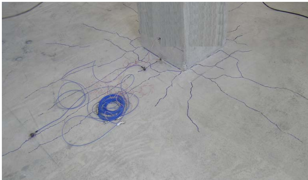
Figure 7.60 Critical crack formed in specimen LG1.0 at 4 in. from column
