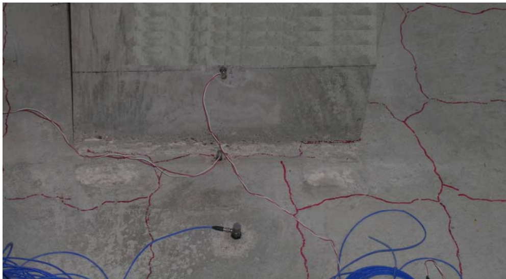
Figure 7.51 Crack at slab-column interface in specimen LR_{ST}G0.5
