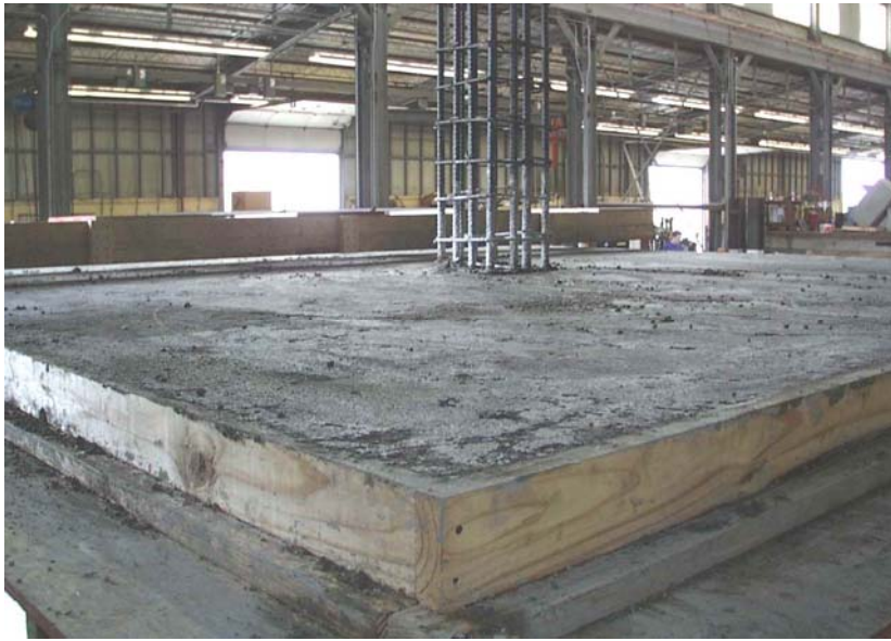
Figure 2.9 Curing of concrete after placement of slab and bottom column
